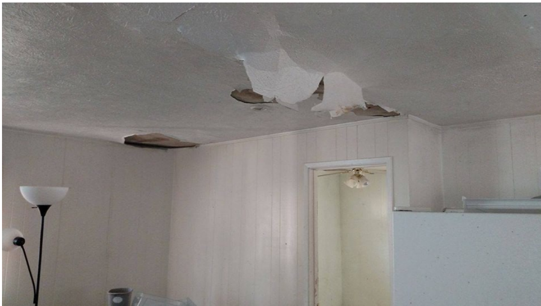
Walking forward from previous photo, then turning southeast; 2 places where ceiling is peeling- some had been pulled down already (& put in trash bags) in this photo.
