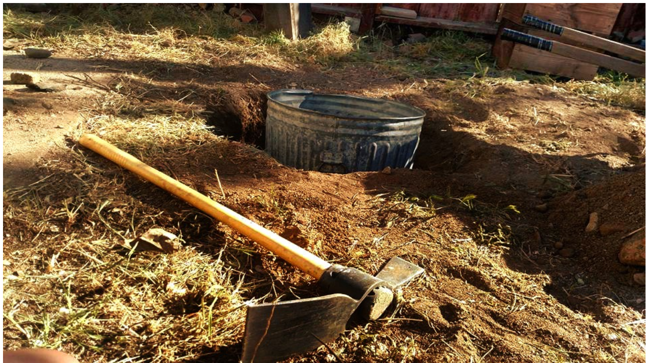
A simple design, "The Burn Toilet" is safe, affordable, & "a drought-wise solution".
