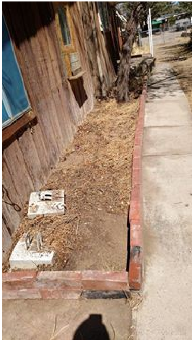
Rebuilt the brick garden bed.
