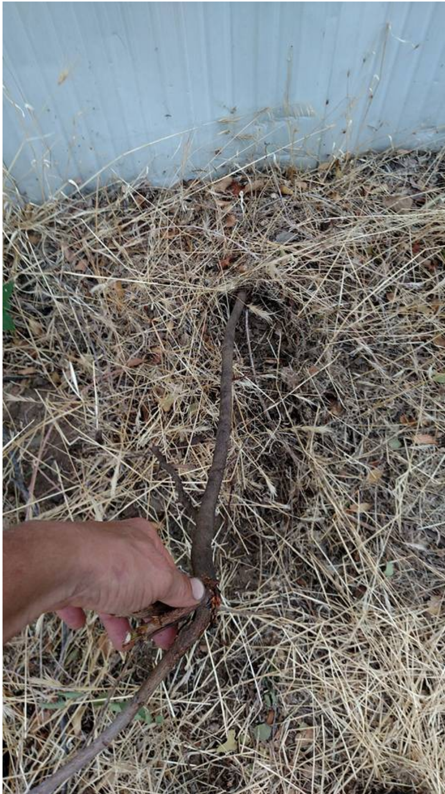
The root systems of the shrubs were endangering the waterlines of the property.
