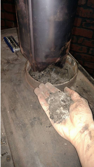
Cleaning out the creosote from the stove pipe.
