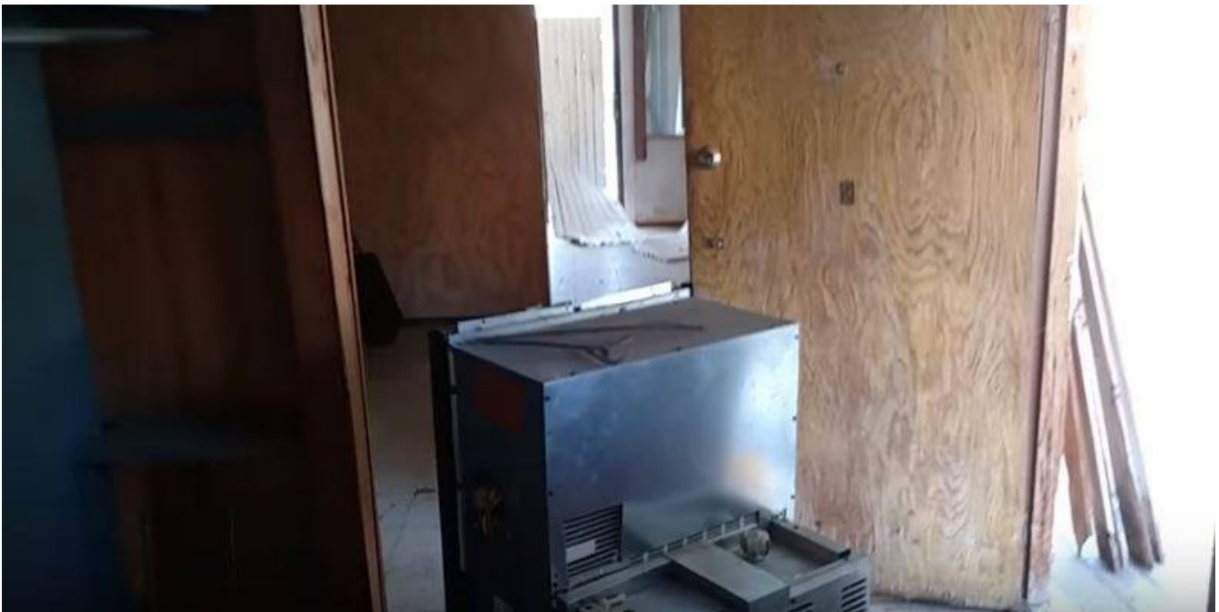
Stepping into the house from front porch, looking to north side of property (front of house).
