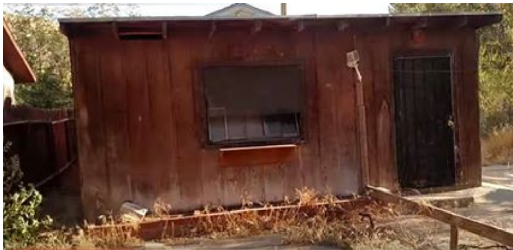
Closeup of rear building as discovered.
