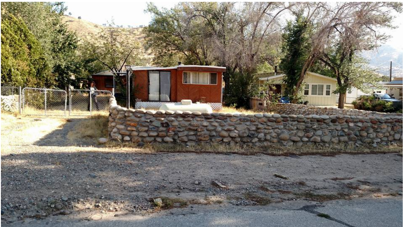
Photo from front of 2232 Commercial Ave. as first discovered.
