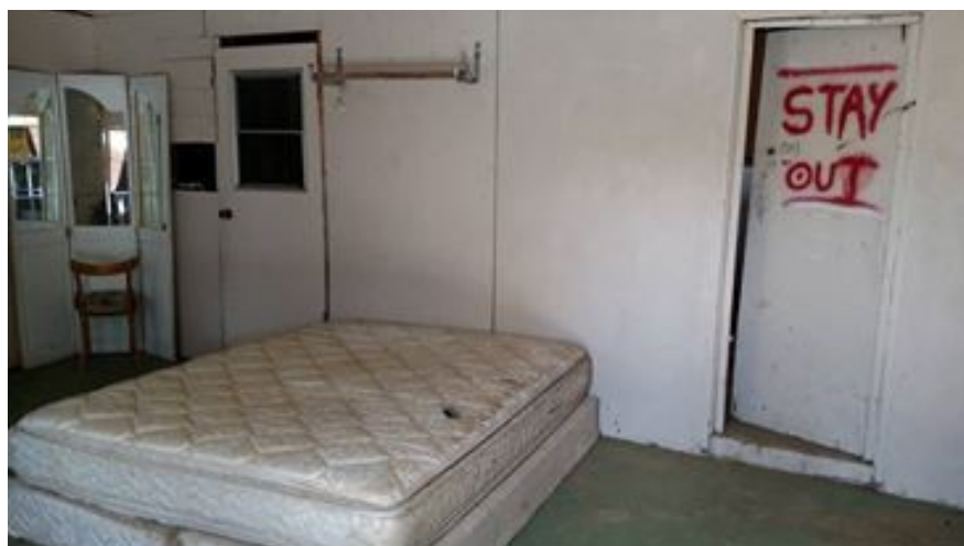
Stepping into rear building (plastic hanging from ceiling removed).
