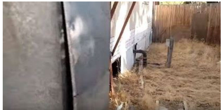
Debris & dried grasses imposing fire hazard on west side of house.
