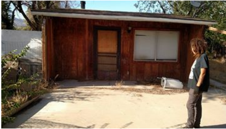
Looking to rear of front building.
