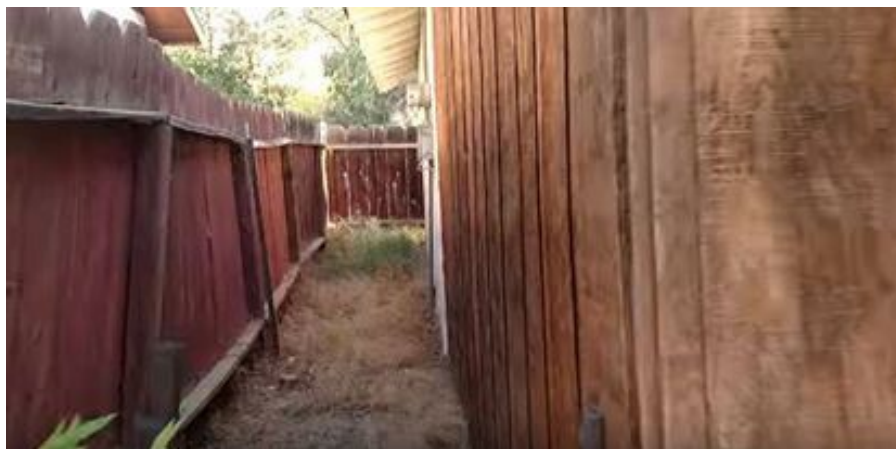
Along east side of rear building as discovered.
