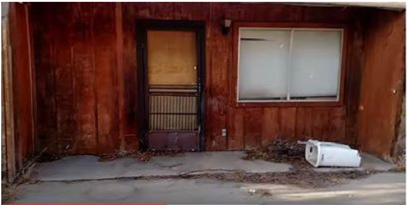
Closeup of rear side of front building.
