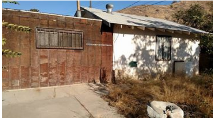
View from west side of rear building as discovered.
