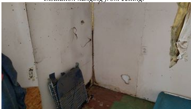
Looking DOWNWARD from previous photo.
