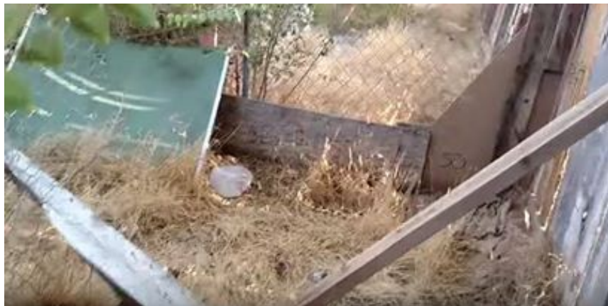
Stepping to the left from previous photo, showing debris & fire hazard on ground as discovered.
