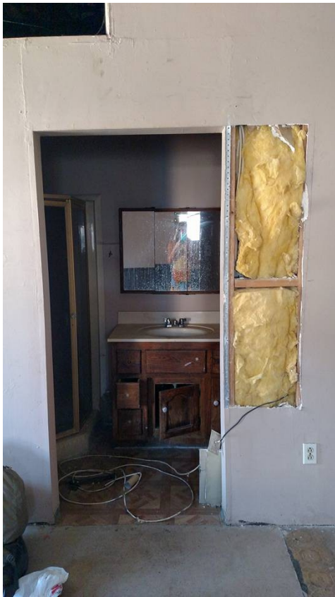
Looking directly into bathroom (floor has been swept now).
